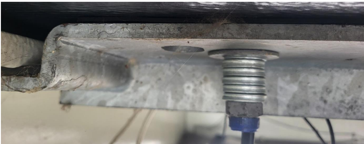
Figure 4.14: Clamping plate at bolt 6
