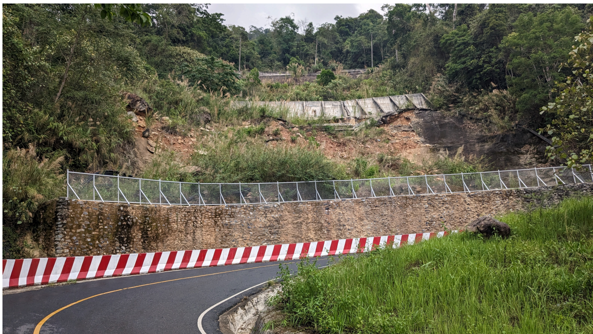
Figure D.5: Large landslide in catchment M43A with different stabilization attempts.
