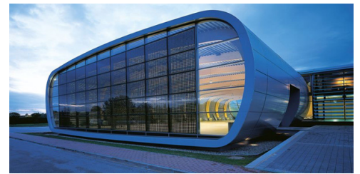
Fig. 22: A reference of a vertical PV façade Company building Tobias Grau, Hamburg (Schaer, n.d.)
