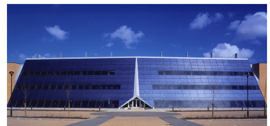
Fig. 34: Reference sloping façade Solar Office Doxford, Sunderland (Studio E Architects, n.d.)
