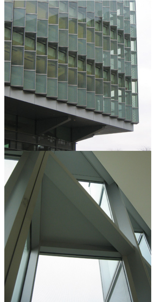
Fig. 25: A reference of a vertical saw-tooth façade. This not a BiPV façade, but it shows the architectural potential Bronx criminal court complex, New York (Seward, 2006)
