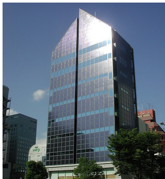
Fig. 6: High-rise hotel, unknown location PV module integrated in the facade composition (Solar Building Tech, n.d.)
