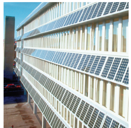
Fig. 26: A reference of a horizontal saw-tooth façade Northumberland building, Newcastle upon Tyne (Roberts, & Guariento, 2009, p. 166)
