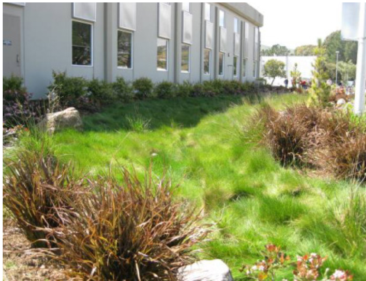
Fig. 2-2-2 Swales of the police department in Brisbane, USA Source: (Hoyer 2011)
