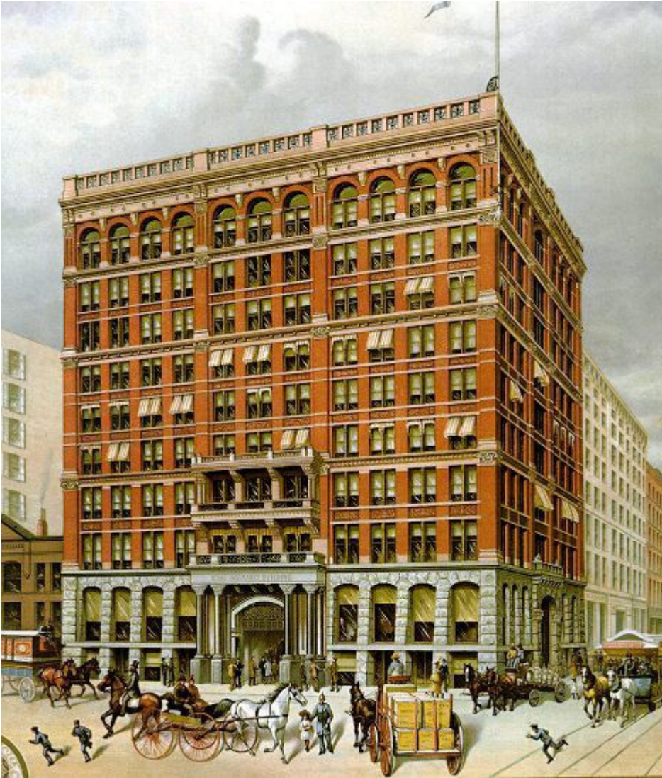
De Home Insurance Building, Chicago (Skyscraper Center, n.d.)
