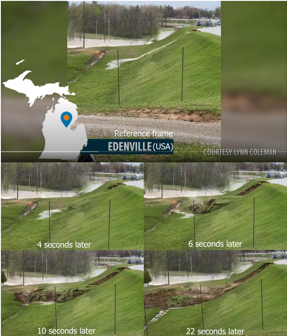
Figure 1.1: Example of flow slide: Edenville dam collapse, USA, May 19th, 2020. Damage included complete destruction of a number of homes, washout of numerous roads and bridges and almost 11000 people evacuated. No loss of life. Videolink: https://youtu.be/Hc3u_CHVHJ8
