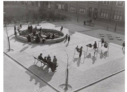
Figure 36. Houses have a watchful eye on the playgrounds and surrounding green spaces (Zaanhof 28-34: De speeltuin, 1952)
