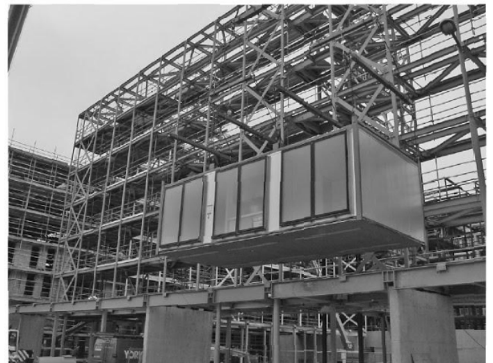
Figure 4.7. Most common dimensions in modular design and partially open-sided modules (source: Lawson, M., Ogden, R., Goodier, C., 2015)
