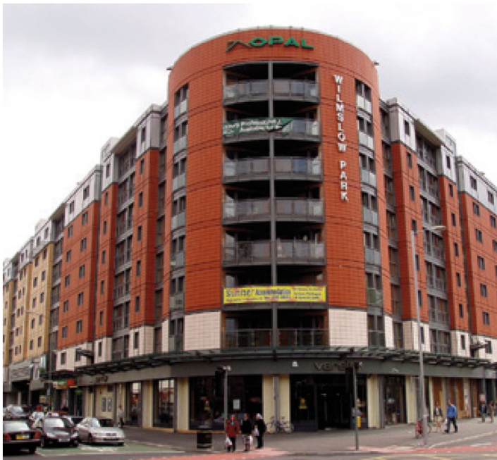
Figure 4.8. Modular construction with support structure and podium structure (source: Lawson, M., Ogden, R., Goodier, C., 2015)
