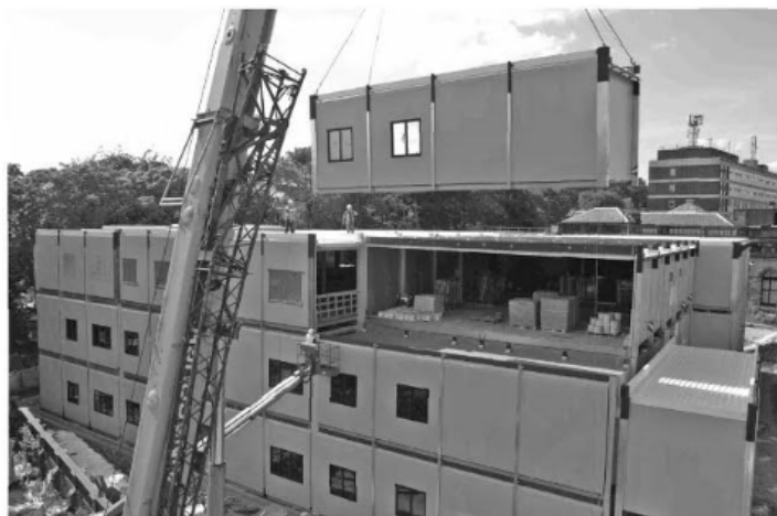
Figure 4.1. 4-sided and open-side modular systems (source: Lawson, M., Ogden, R, Goodier, C.,
