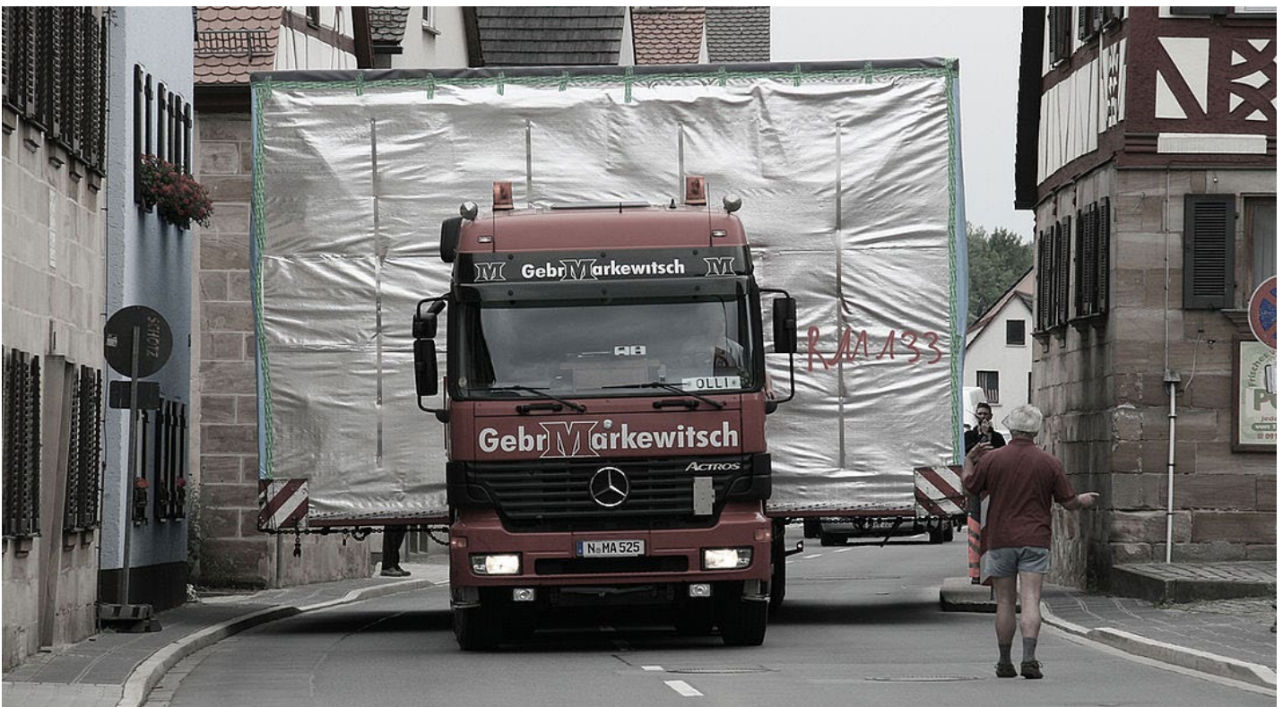
Figure 5.21. Transportation of the module. ( Cadolto.com )
