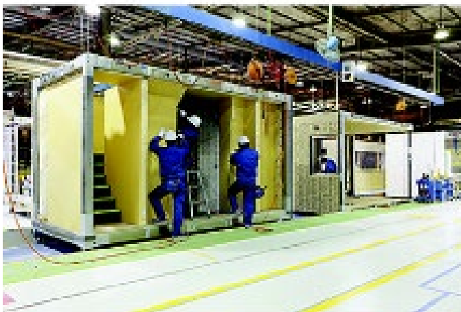
e) Equipping of unit frame structure with finishing components
