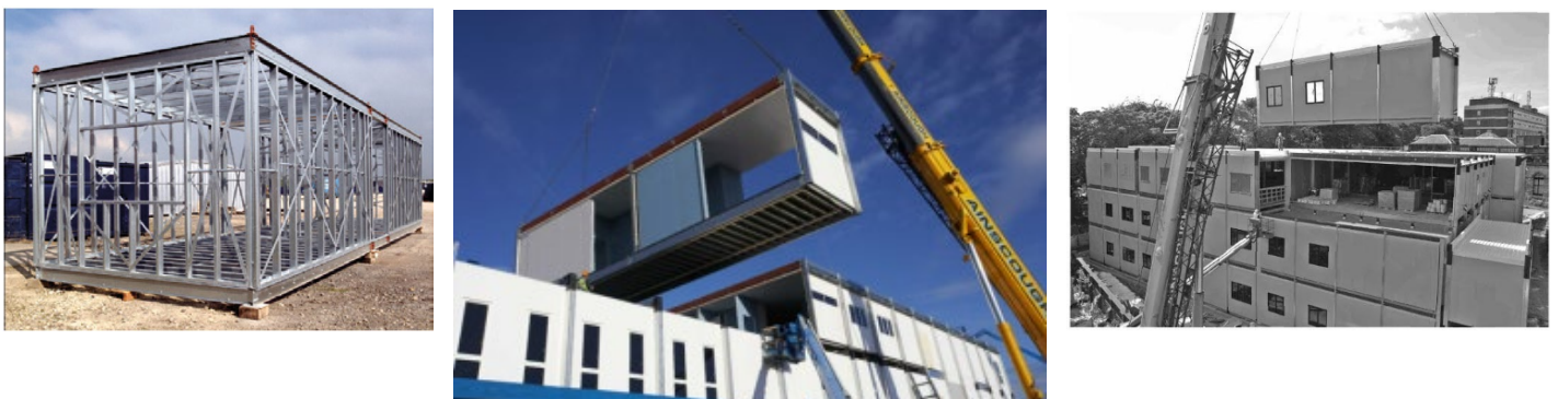
Figure 4.4. 4-sided, partially open-sided and open-sided modules (source: Lawson, M., Ogden, R, Goodier, C., 2015)
