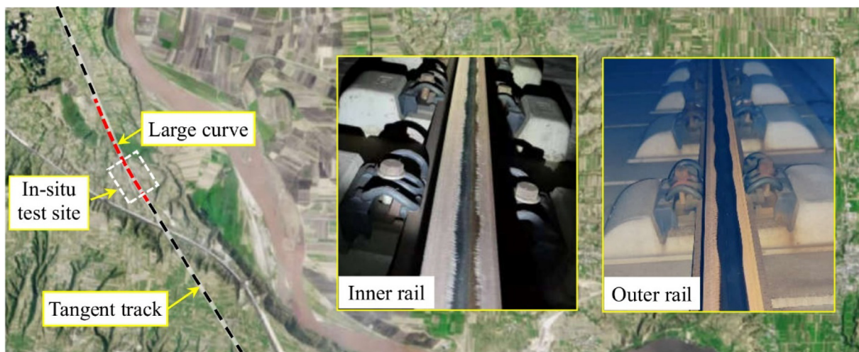
Fig. 7. Rail corrugation on the large curve of the HSR track B.
