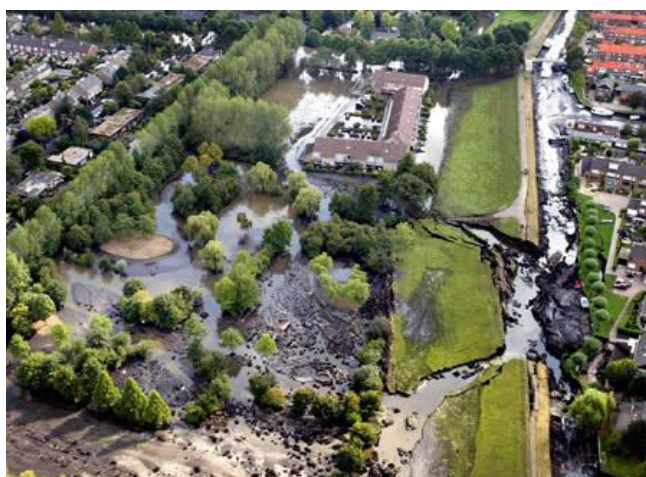
Figure 1: Horizontal failure of the Wilnis peat dyke (Van Baars 2005)
