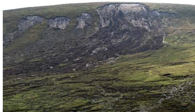
Figure 2: Peat slope failure in Ireland (Long and Jennings 2006)
