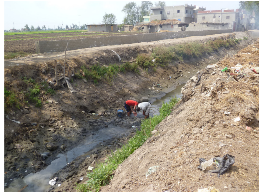
^ Farmers building an obstacle to keep water in Nile Delta, (When canals dry up farmers sometimes build small earth obstacles in order to raise the water level near the inlet of their pump station. François Molle, 2017, via Flickr
