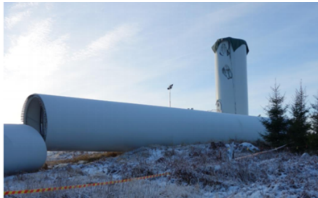
Figure 1-3: The collapsed Lemnhult wind tower with the bottom part anchored to concrete base [9].
