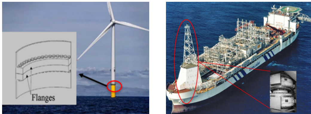
(a) Foundation pile attached to the turbine support structure by means of a bolted ring flange connection [6]. (b) Critical bolted connection in an FPSO turret swivel system [7].
