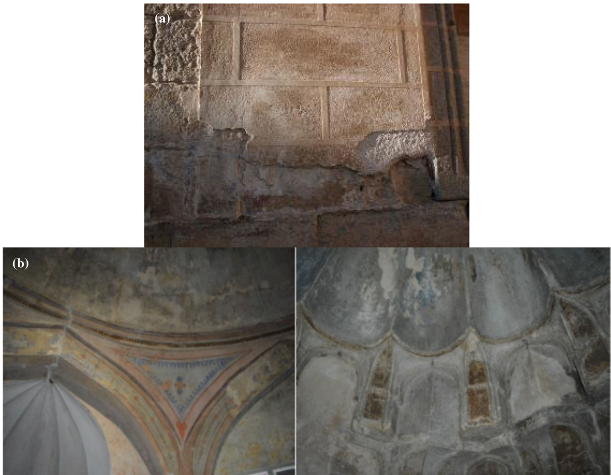
Fig. 3 a Durability of air lime render imitating stone over stone masonry in Évora Cathedral, in Portugal (seventeenth century); b Interior of Pasa Hamam, Thessaloniki (1530 AD), with well-
