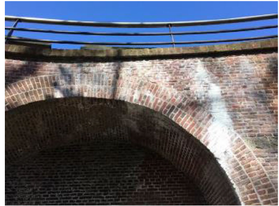
Fig. 33 Arch section in the masonry of the motte castle of Leiden, after reconstruction of the section
