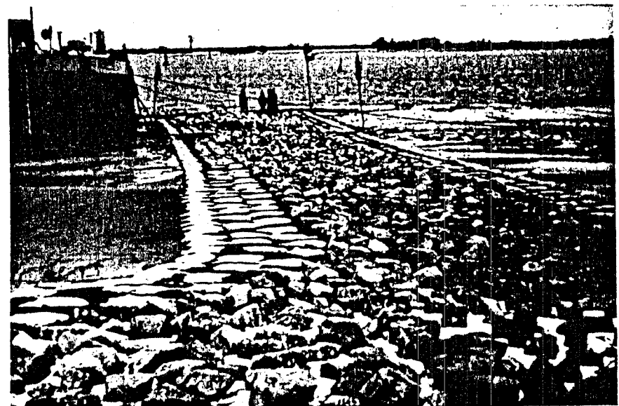
Fig. 11 Groin under construction
