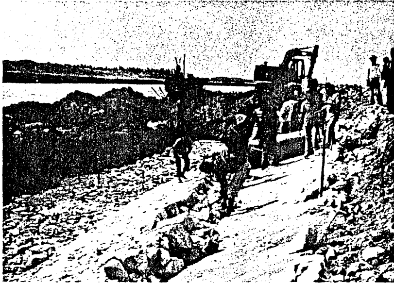
Fig. 7. Hand-placing of riprap direct onto the geotextile.
