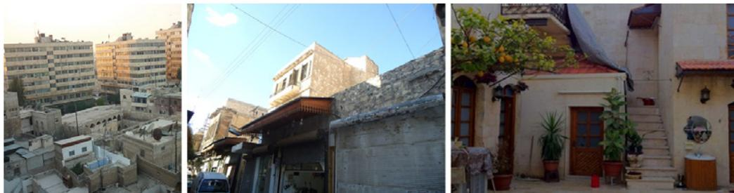
FIG. 3 Architectural anomalies and changes in functions made by inhabitants before the Syrian Civil War: adding rooms on the first floor, adding additional floors and changing the residential functions to commercial one, and adding a toilet and a bathroom in the courtyard (left to right). Source: author – field work 2010.
