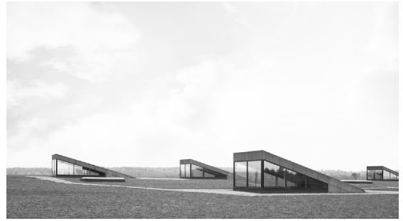
8.1.15 Solrødgård Water Treatment Plant
