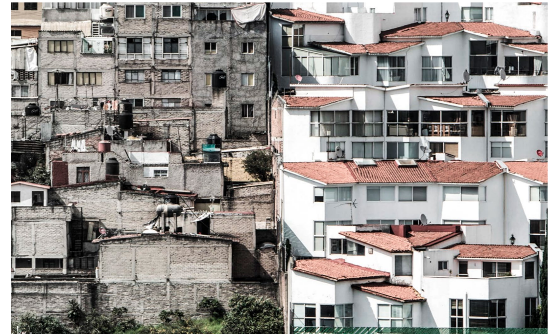
Figure 5. Source: UNEQUAL SCENES, 2019. The image depicts Spatial Fragmentation, high income and low income developments in the same place
