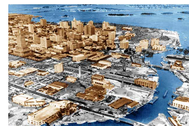
1970s Fewer public space accessible to the river Many alien settlers went to riverside neighborhood The downtown formed near the downstream river
