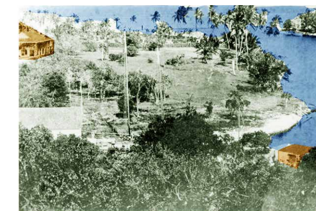
1894 Before Florida railway was built Miami River not exploited Natural river bank & vegetation
