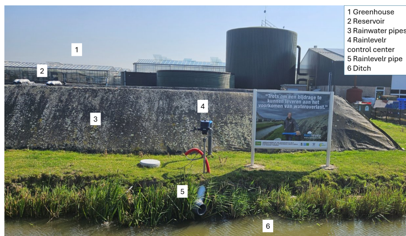
Figure 1.7: Rainlevelr setup at Ammerlaan Growers (Adapted from Picture: Sabine van Esch).
