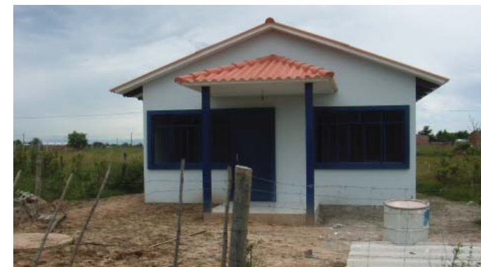
Fig. 5.14 "Cheap" housing 12km from the city's centre
