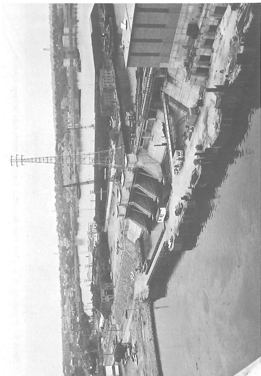
Figure 8. Providence, R. I. - Fox Point Hurricane Barrier Showing Tainter Gates
