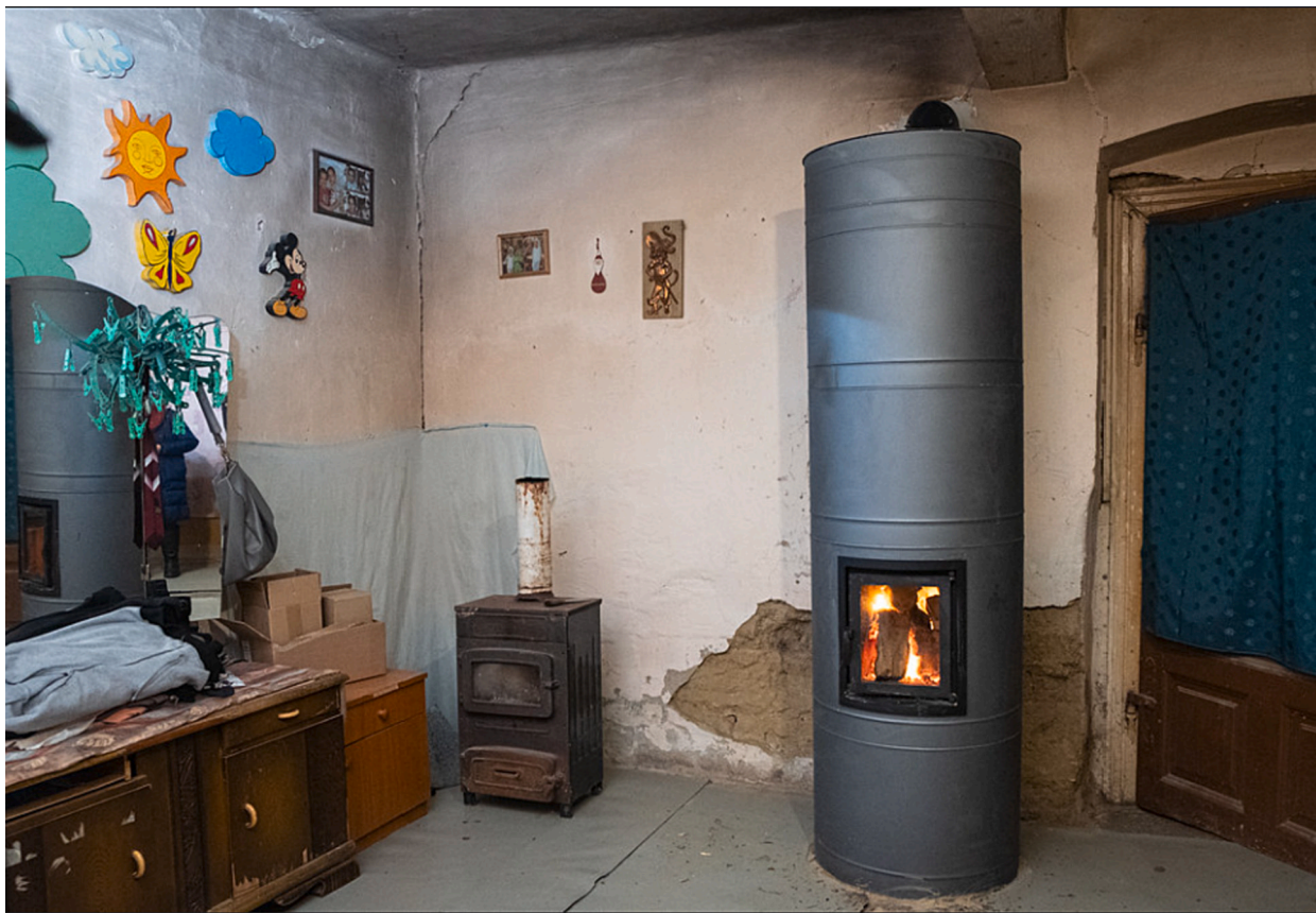
Fig. 4. Replacing an old fuelwood stove (on the left) with a new one in Hungary. Source: [101].
