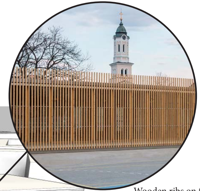
Wooden ribs on facade
