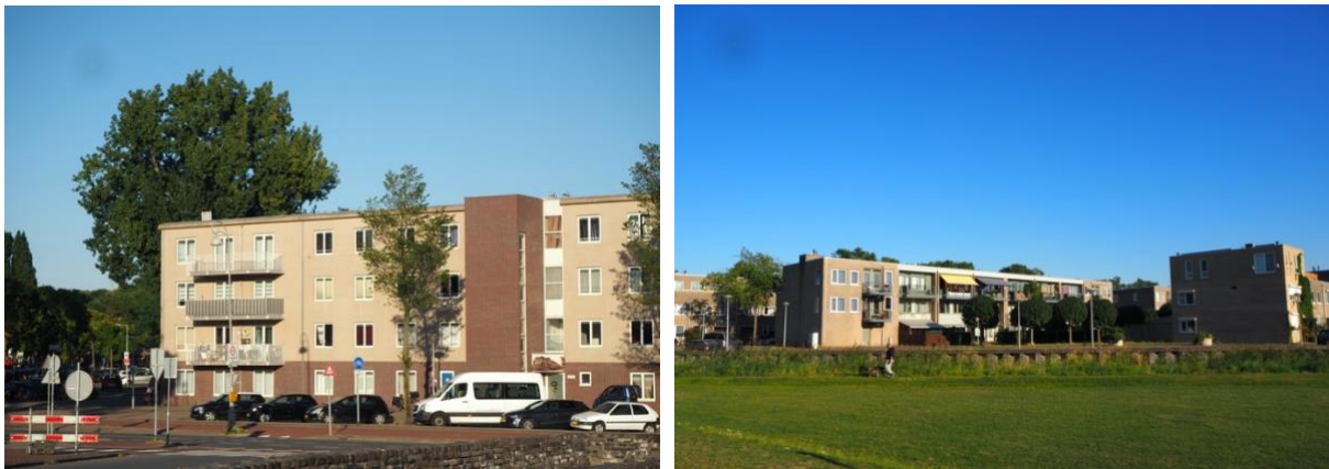
Figure 8. 70s buildings IJplein/Vogelbuurt
