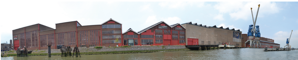
Figure 6. RDM campus. Source: Paolo De Martino.
