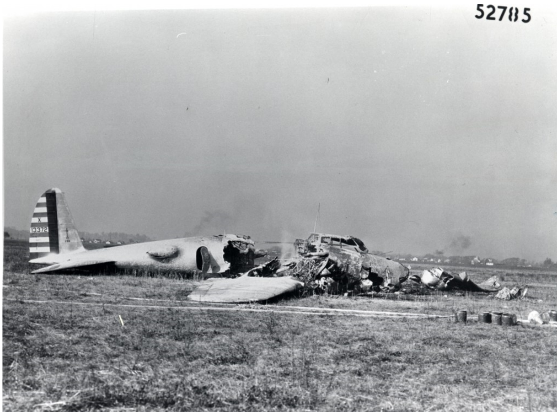
Fig. 1 Side view Model 299 after the crash during evaluation exercise [4].
