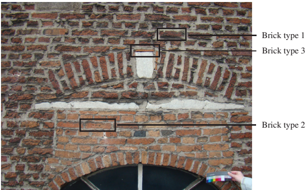
Figure 7: Inspection area B4.
