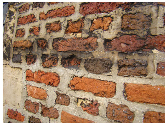
Figure 12: Upper part cleaned with steam cleaning, lower part cleaned with wet-jet abrasive cleaning.
