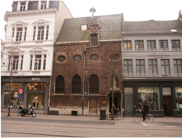
Figure 1: Main façade of the Schoenmakerskapel and its immediate surroundings, 2011.
