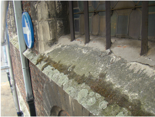
Figure 4: Windowsills in natural lime stone with an additional layer in cement mortar.
