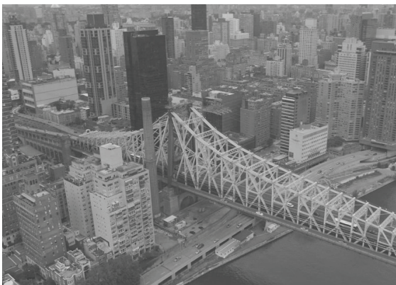
4.1.6 Ed Koch Queens boro bridge entry node
