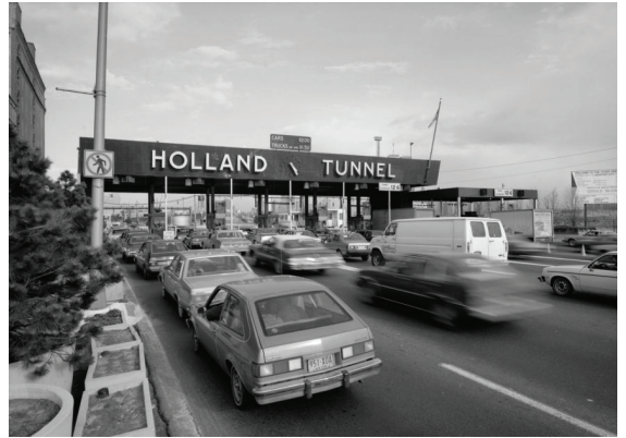
4.1.5 Toll entries at the Holland tunnel
