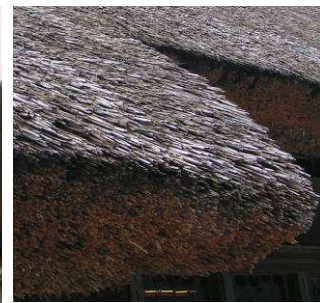
Picture 7-1 Close up of a Thatched Roof
