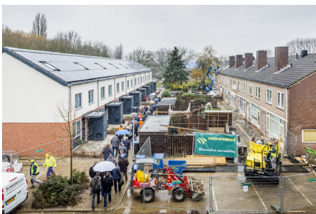
Figure 19: Project stroomversnelling in progress (flickr.com).
