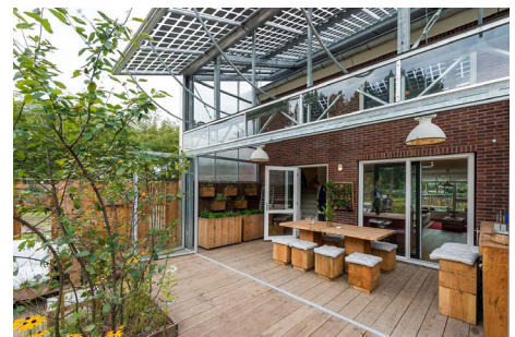
Figure 22: The greenhouse extension of the Prêt-à-Loger (thegreenvillage.org).
