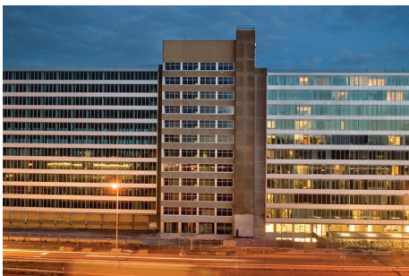
Figure 12: Before and after facades of the GAK-gebouw in Amsterdam (rufusdevries.nl).
