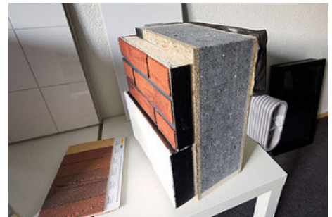
Figure 20: A detailed model of the prefabricated facades (flickr.com).
