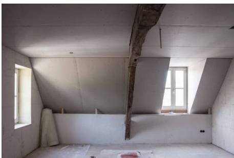
Figure 13: An internally insulated attic (bedi.nl).
