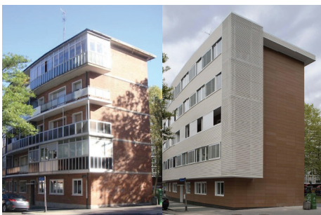
Figure 14: Before and after facades of an externally insulated building (buildup.eu).
