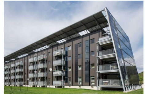
Figure 15: New elements were added to the building to increase space, improve indoor climate and produce electricity (buildup.eu).
