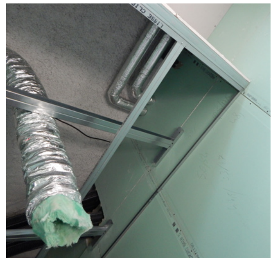
Figure 18: Soffit to adapt to existing windows (own picture)
