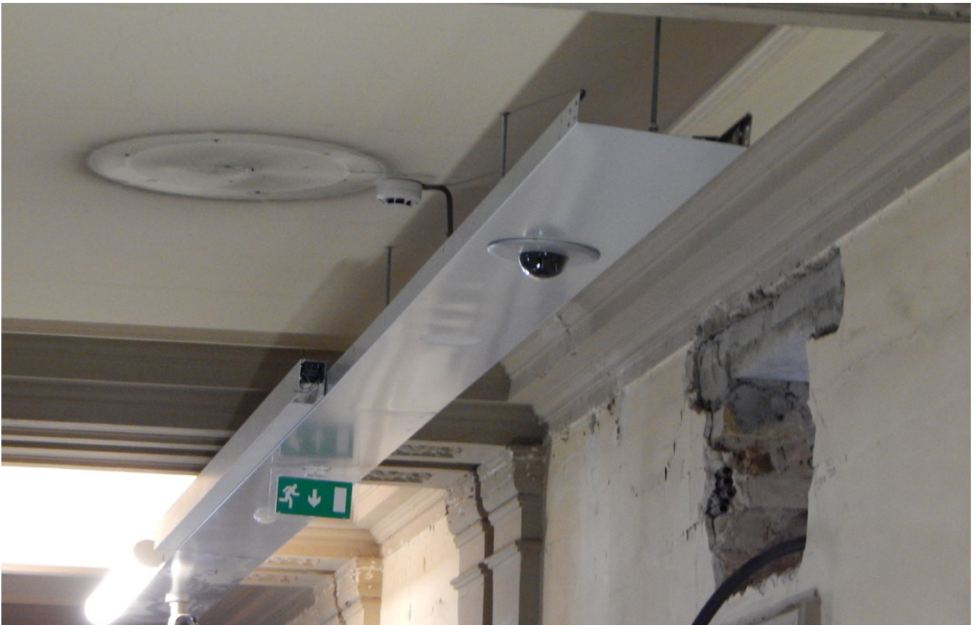
Figure 24: The cable rail prototype with two lighting rail variants and several installations including a smoke detector on the ceiling. (own picture)
