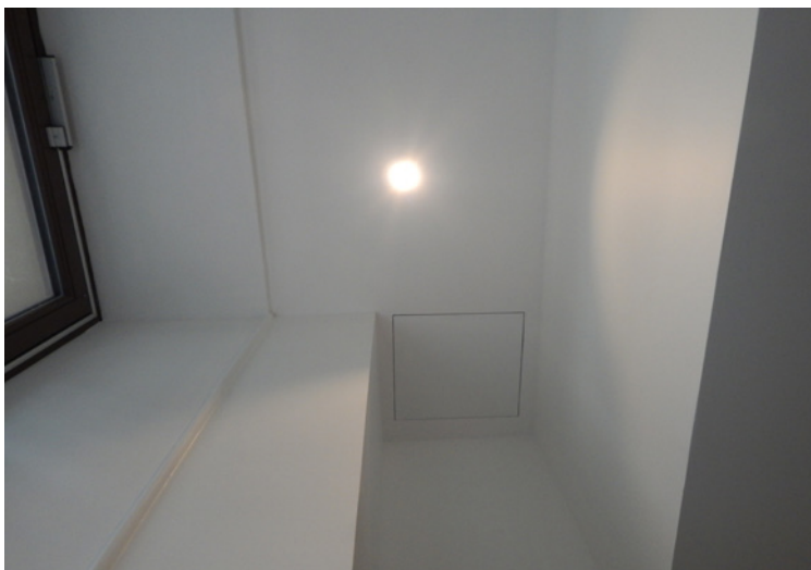
Figure 18: Soffit to adapt to existing windows (own picture)
