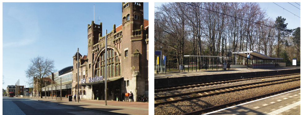
Fig. 7.28 Haarlem station, which is regionally and locally well connected (left), and Sandpoort Noord station, a poorly connected train station with only a ticket machine (right)
