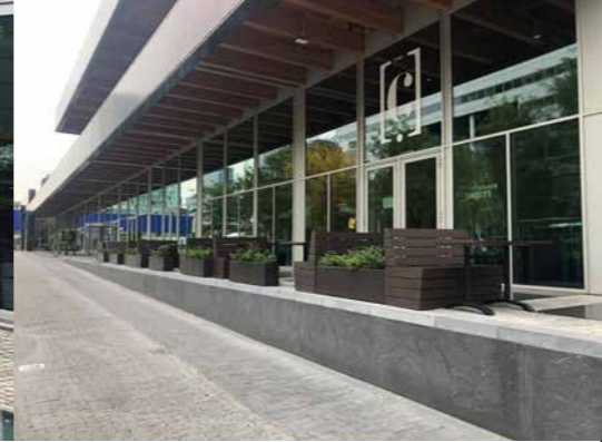
Figure 4.21 (upper left) Plinth of CIRCL from Mahlerplein side (own photography).
