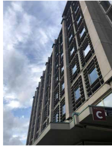
Figure 4.84 The façade at Weena side (own photography).
