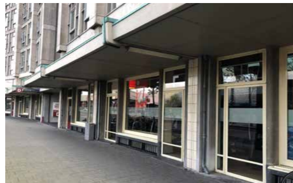
Figure 4.79 Plinth at the north side of Groot Handelsgebouw (own photography).
