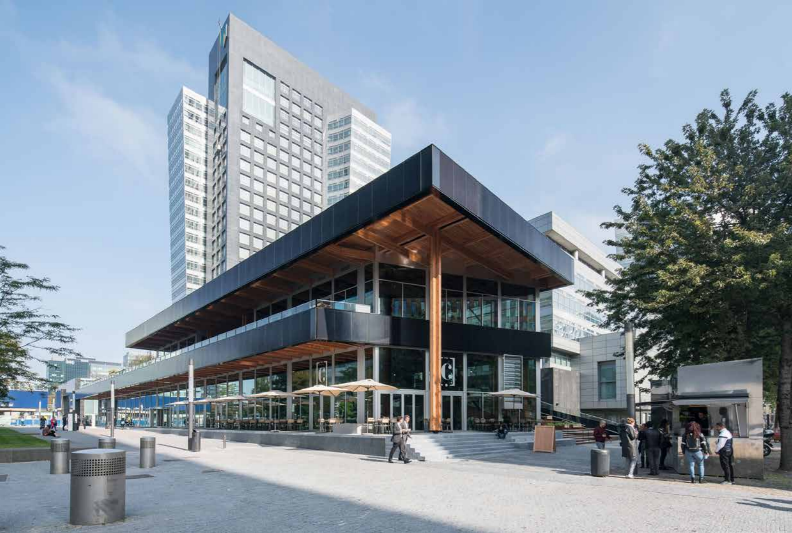
Figure 4.8 ABN AMRO CIRCL building (photo by van Duivenbode, O.)
