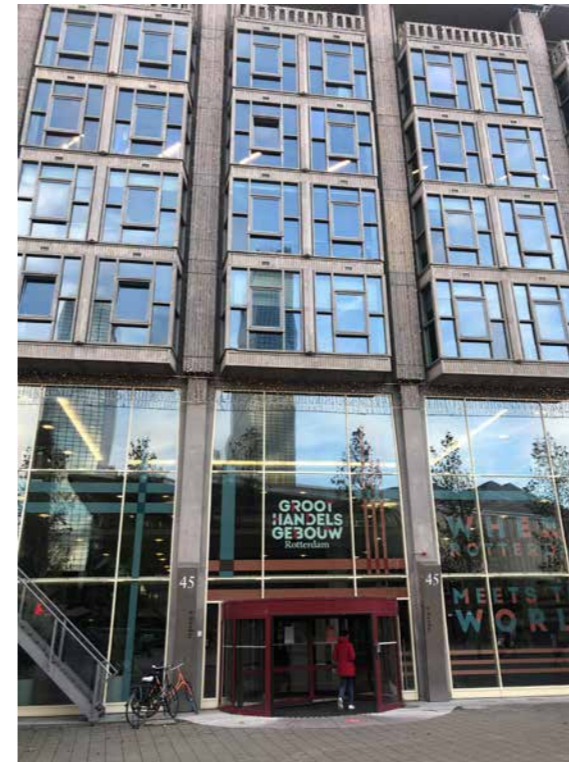
Figure 4.80 Plinth of the main entrance (own photography).
