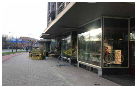
Figure 4.78 General plinth of Groot Handelsgebouw at Weena side (own photography).
