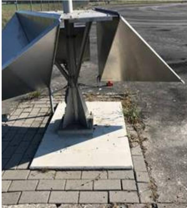
Figure 4.6: Potential lateral forces working on the concrete base plate of the platform of station **KOLH**, e.g. due to thermal expansion of the pavement structures. After an intervention on 26 June 2020, when a buffer zone was established, the station stabilized (Piëning, 2021).
