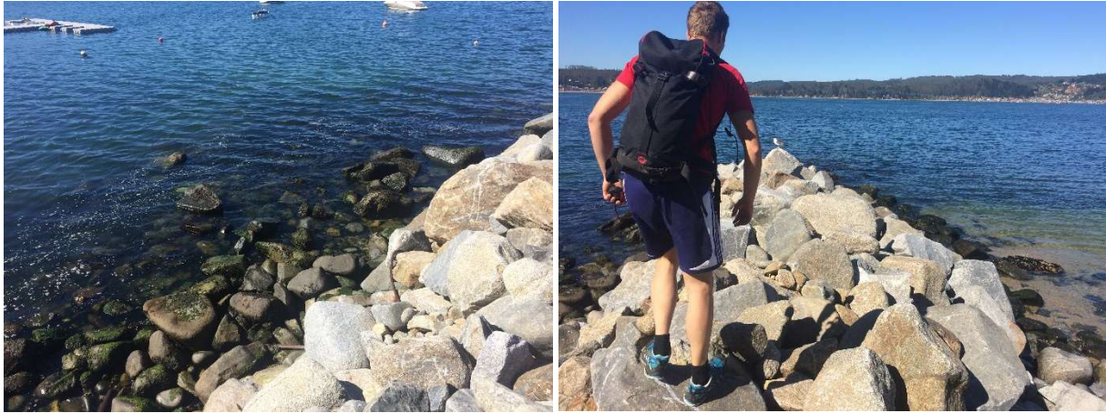
Figure 1-11: Breakwater to the North of jet ski jetty
