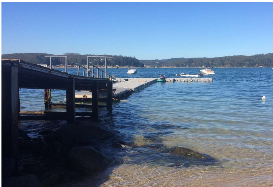
Figure 1-10: Jet ski floating jetty
