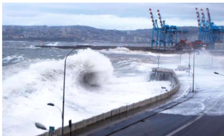
Figure 2-14: Winterstorm August 2015, at the port side of Valparaíso (Winckler, 2016).
