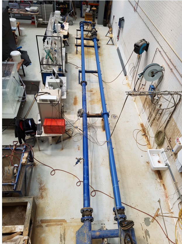
Figure I.4: Top view of the horizontal part of the slurry loop
