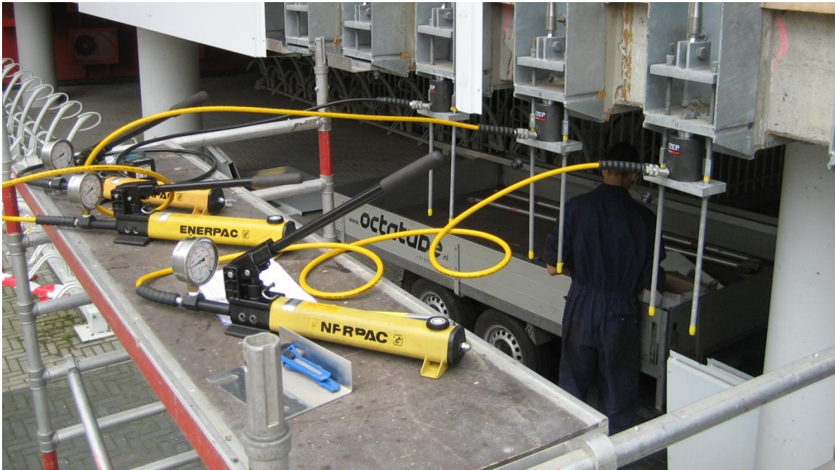
Figure 194 Hydraulic jack with pressure gauge (Peter van de Rotten, 2013)
