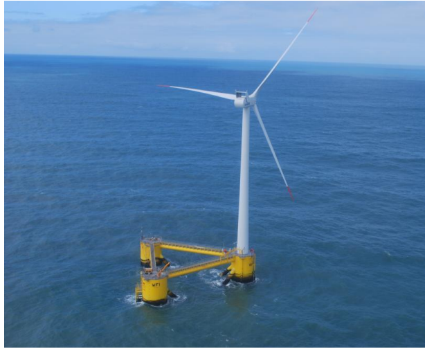
Figure 1-2: The WindFloat concept [4]
