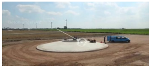
Figure 4.1: A recently finished wind turbine foundation
