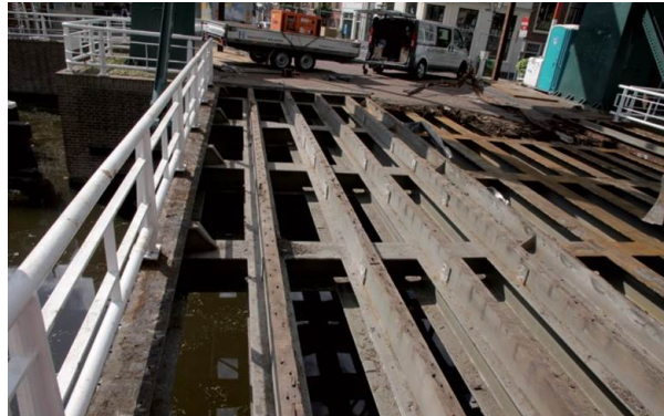
Figure 1.1: Renovation bridge deck of Marebrug, Leiden
