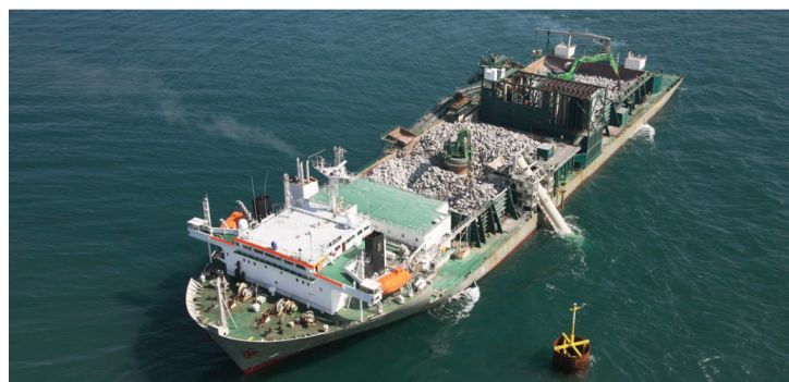
Figure E.7: The Seahorse, one of the Fall Pipe Vessels (FPV) of Boskalis' fleet, during installation of a rock layer.
