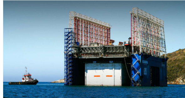
(b) Launch and towage of the caisson to intermediate storage.
