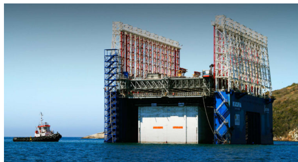
Figure D.4: Floating caisson-building dock Kugira deploying a caisson. [Image: Acciona]
