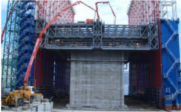
(a) Caisson fabrication at a floating caisson-building dock.
