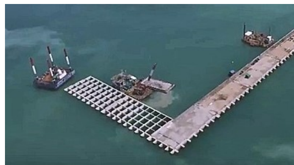
(f) Installation of the caisson, including the ballasting and positioning.
