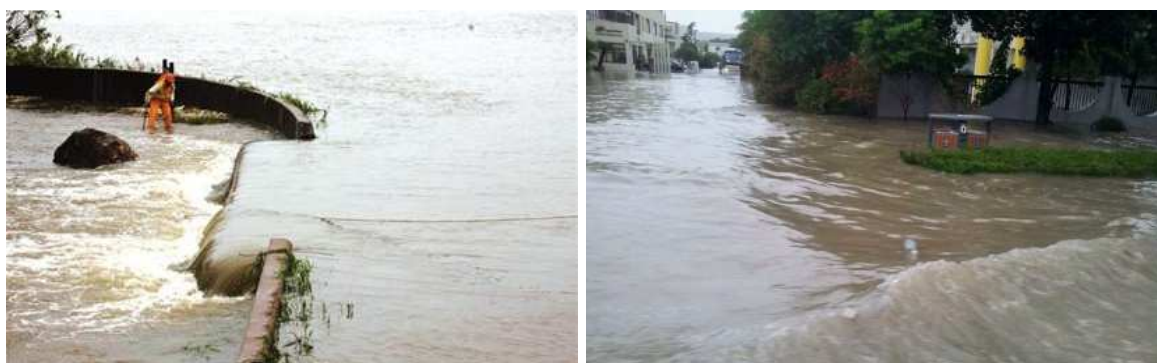
Fig.2. 11 Floodwall breach in the upstream of the Huangpu River in October of 2013, which led to inundation in adjacent farmland and residential buildings 3
