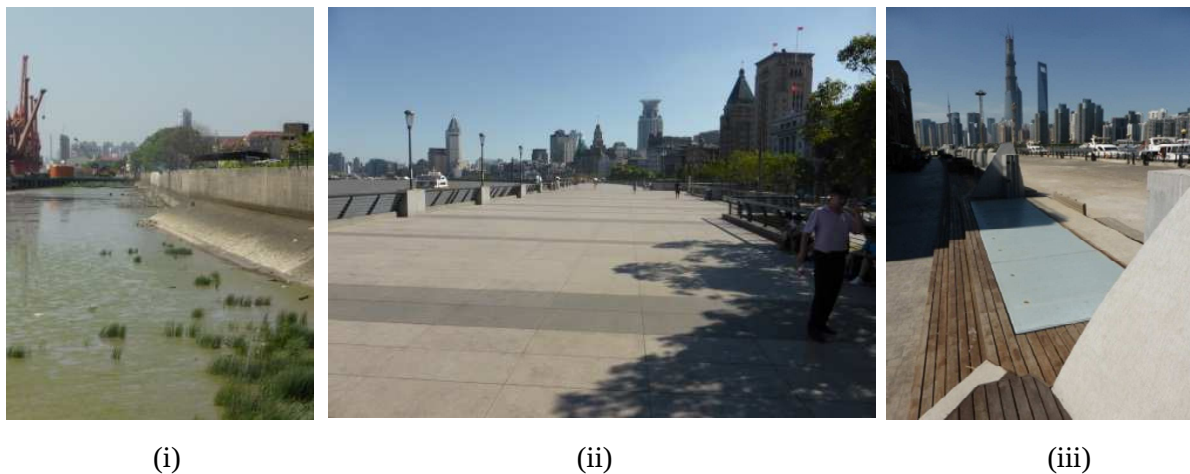
Fig.2. 18 Field observation of floodwall along the Huangpu River in 2013 (i) floodwall with revetment (ii) Bund sight-seeing floodwall (iii) small flood gate in glass
