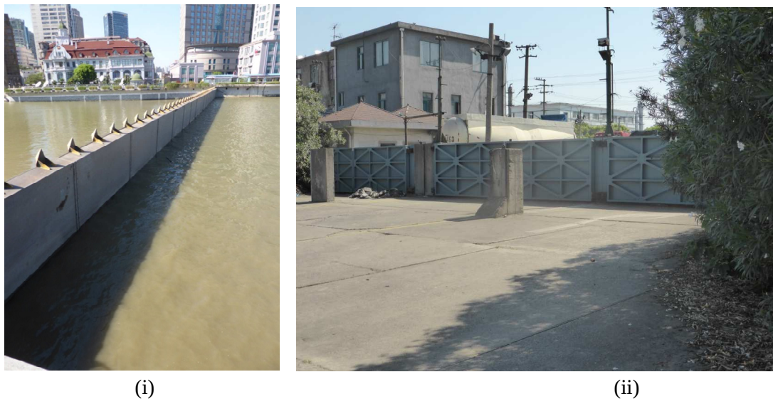
Fig.2. 21 (i) Suzhou Creek gate and (ii) typical floodgates in Shanghai
