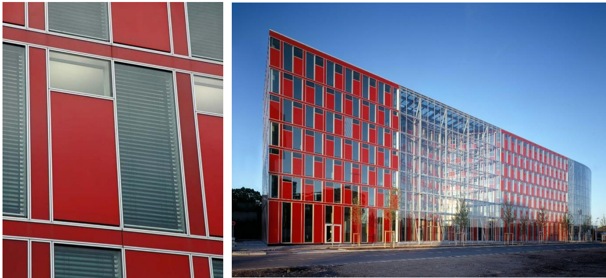
Figure 4.1: Facade module of the Capricorn Haus (Left) and the overall facade pattern (Right).
