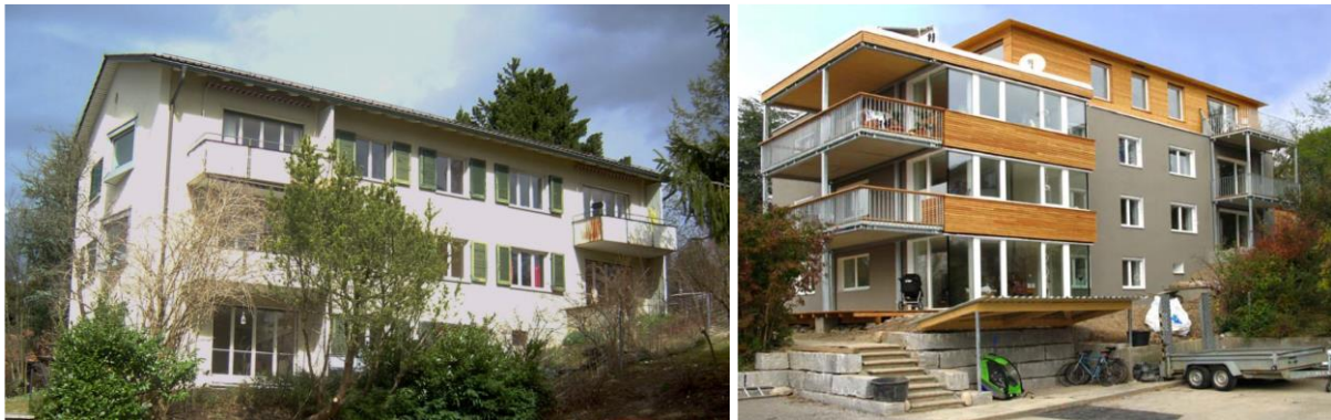
Figure 4.3: Photos of the apartment before (Left) and after (Right) the renovation project.
