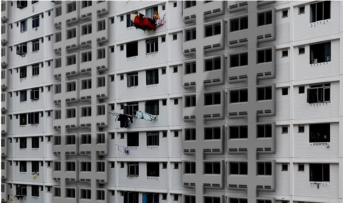
Figure 5.29: A visualisation of what the facade modules would look like without the facade-located ETC tubes.
