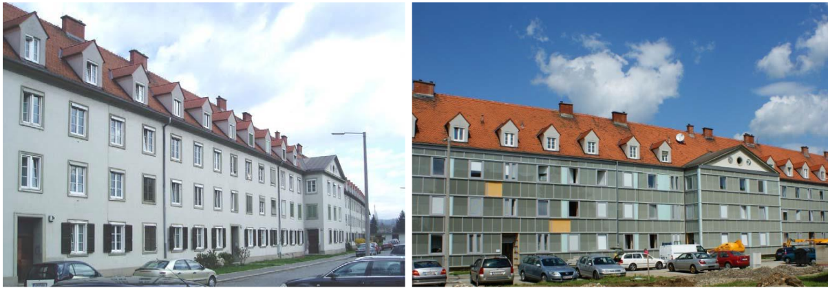
Figure 4.6: Photos of the building before (Left) and after (Right) renovation.
