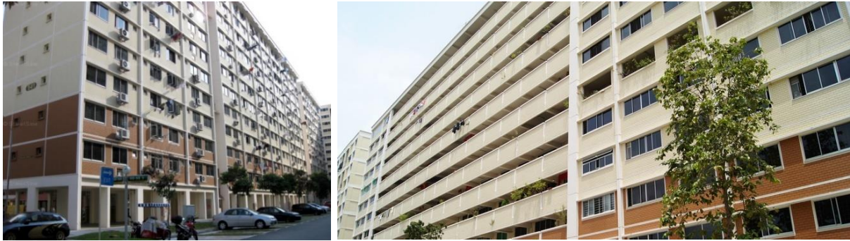
Figure 2.24: The North facade of the building (Left) and the South facade (Right).
