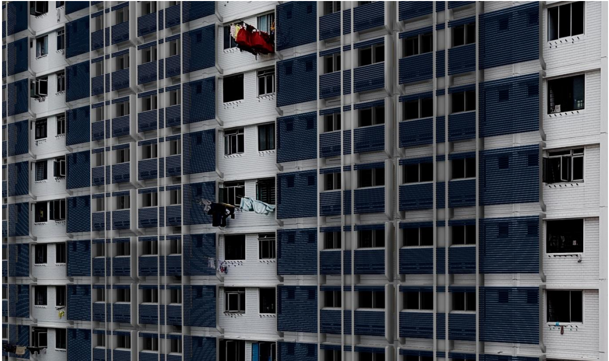
Figure 5.27: A visualisation of the array of facade modules on the existing building.
