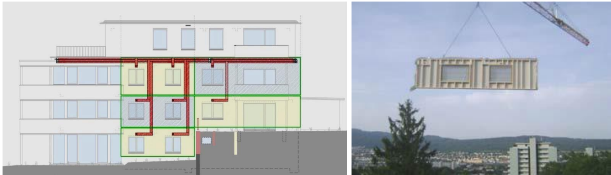
Figure 4.5: Diagram showing the ventilation distribution (Left), and a photo of the prefabricated 3 x 10 m facade module being lifted to be mounted during construction (Right).
