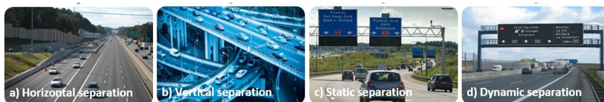
Figure 2-1. Types of traffic flow separation; horizontal (Watts, 2013), vertical (Schnabel, 2015), static (van Reeken, 2010), dynamic (SWARCO, 2015)
