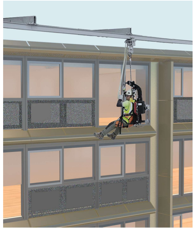
Figure 82. Electrical duct and façade maintenance procedure with a ropeclimber and a substructured at the top of the building
