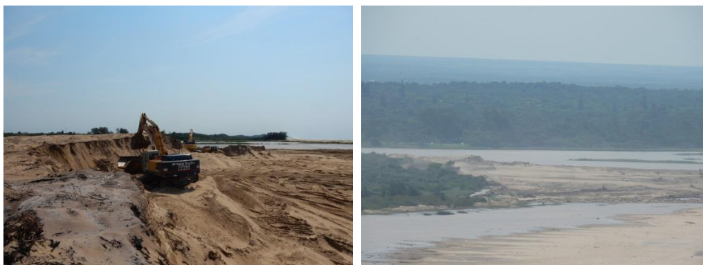
Figure 5.28: Photos of dredge spoil removal in St Lucia Estuary
