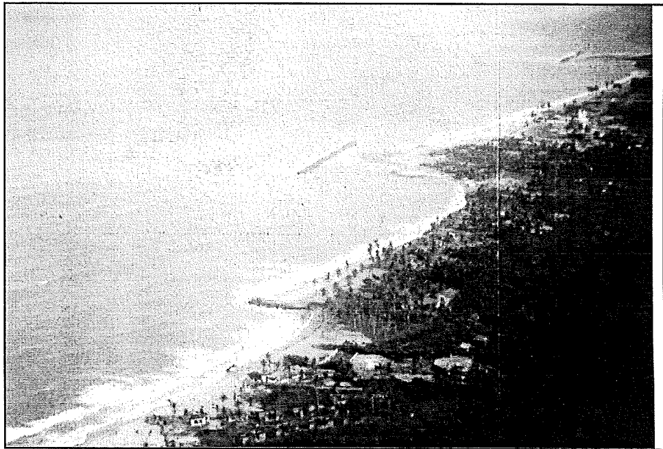
P -3 : Most northward breakwater and short groyne
