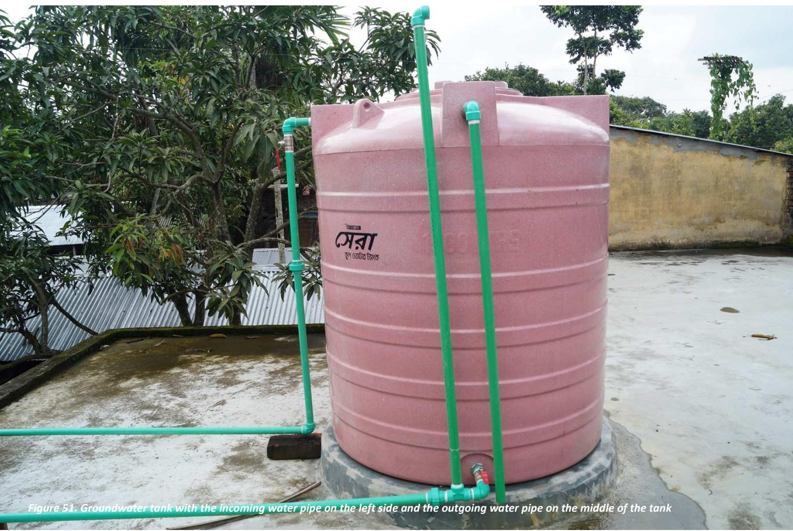
Figure 51. Groundwater tank with the incoming water pipe on the left side and the outgoing water pipe on the middle of the tank
