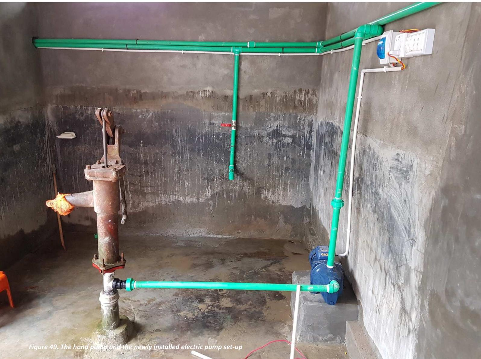
Figure 49. The hand pump and the newly installed electric pump set-up
