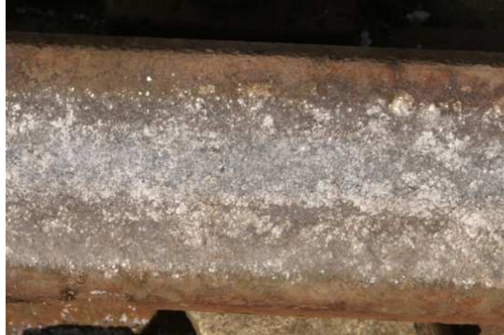
Fig. 3A.16. Photograph of the top of a rail after four locomotive wheel passages over a sanded track.
