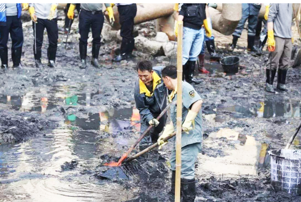
洗河 Dredging The River
